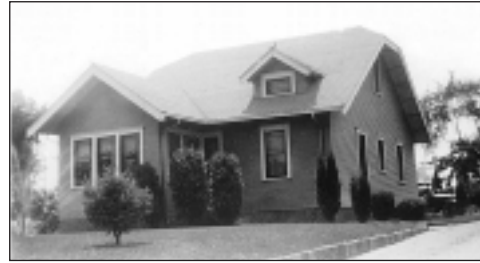
Killian and Bertha Feser new Wayzata home, 1926. It's still on highway 12, in town just east of the grave yard
